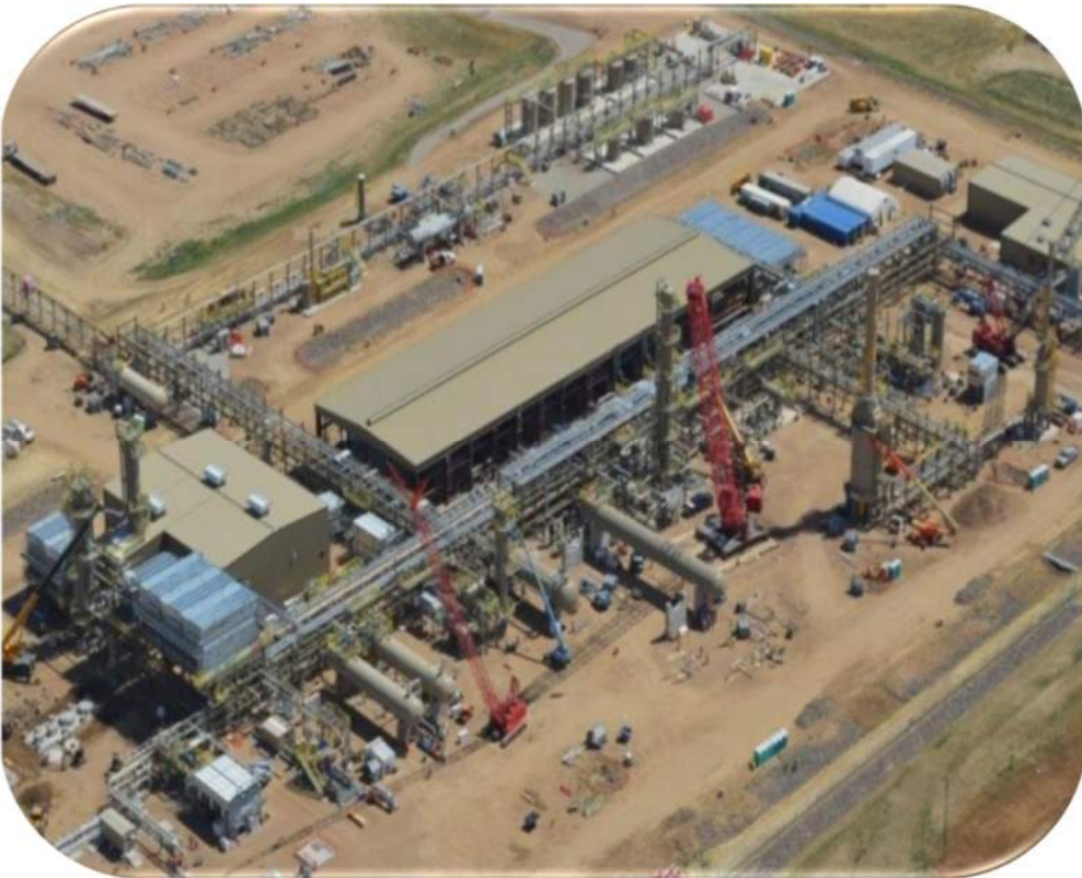
DCP O'Connor Gas Plant CCS, Kersey Colorado
