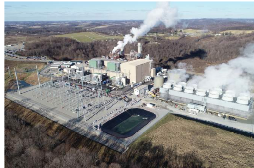
Tenaska Westmoreland Generating Station – Combined Cycle
