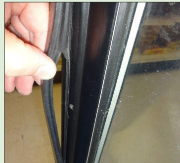
Figure 5: Inspecting gaskets and seals can reveal potential losses in efficiency.
