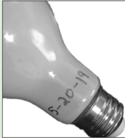
Figure 2: Writing the date that the light bulb was installed on the base of the light bulb will help you keep track of when each light bulb was installed.
