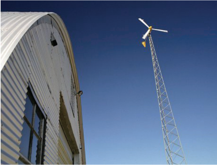
Small wind turbines, like this grid-connected Bergey 10 kW Excel in Scott City, Kansas, can provide supplemental power for farms and ranches. Excess power is fed back into the utility grid. (Photo by Warren Gretz, NREL Staff Photographer.)
