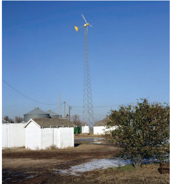
A grid-connected Bergey 10 kW Excel in Scott City, Kansas (Photo by Warren Gretz, NREL Staff Photographer.)
