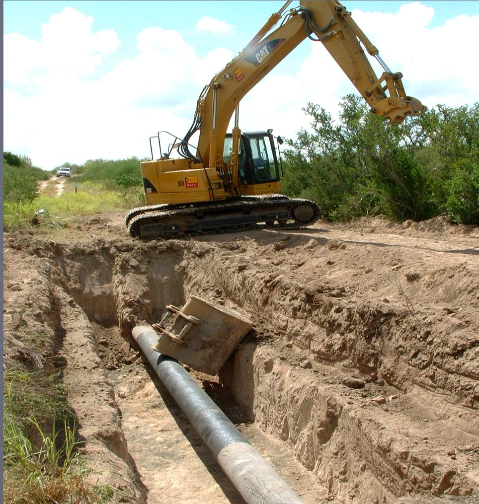
► After management and safety were on scene it was determined that the Track Hoe was equipped with a hydraulic quick coupler attachment for the bucket. This type of equipment is common in the utility excavation business, but not so common in the pipeline excavation business. After interviews were conducted, it was revealed that no one onsite had prior knowledge nor training about this feature.
